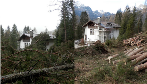
Figure 1 Left: Centre of Studies for the Alpine Environment (Belluno, Dolomites, Italy) on October 30, 2018, on the day after the event. Notice fallen trees on the roof of the building and part of the damages done in its vicinity. Right: Same position two months later (January 4, 2019), with the first restoration works (Photographs: Roberto Menardi).
